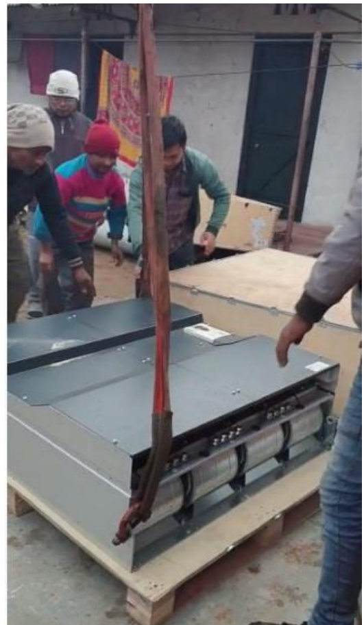
Variable Frequency Drive (VFD) under installation
