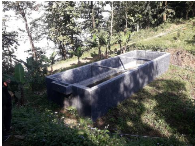
Sedimentation Tank at Lirmen Village
