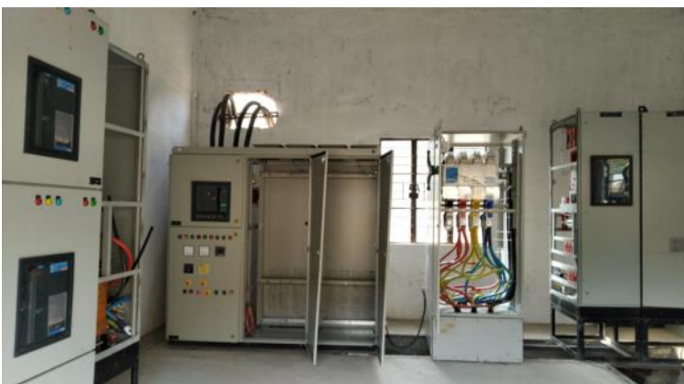
Variable Frequency Drive (VFD) under installation
