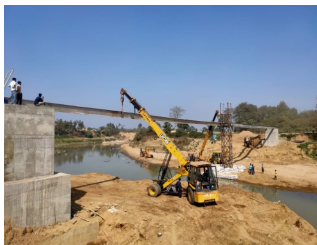
Ongoing Howe Truss bridge construction for carrying Dimapur Town sewage across Dhansiri river
