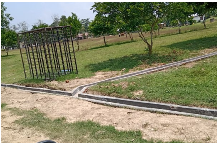
Waste Collection Pit, Soak Pit and Drainage constructed under Solid & liquid Waste Management Works
