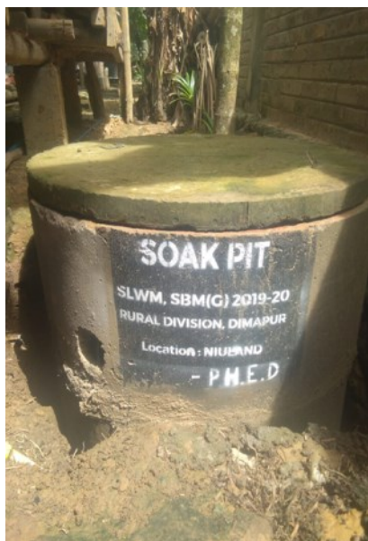
Waste Collection Pit, Soak Pit and Drainage constructed under Solid & liquid Waste Management Works
