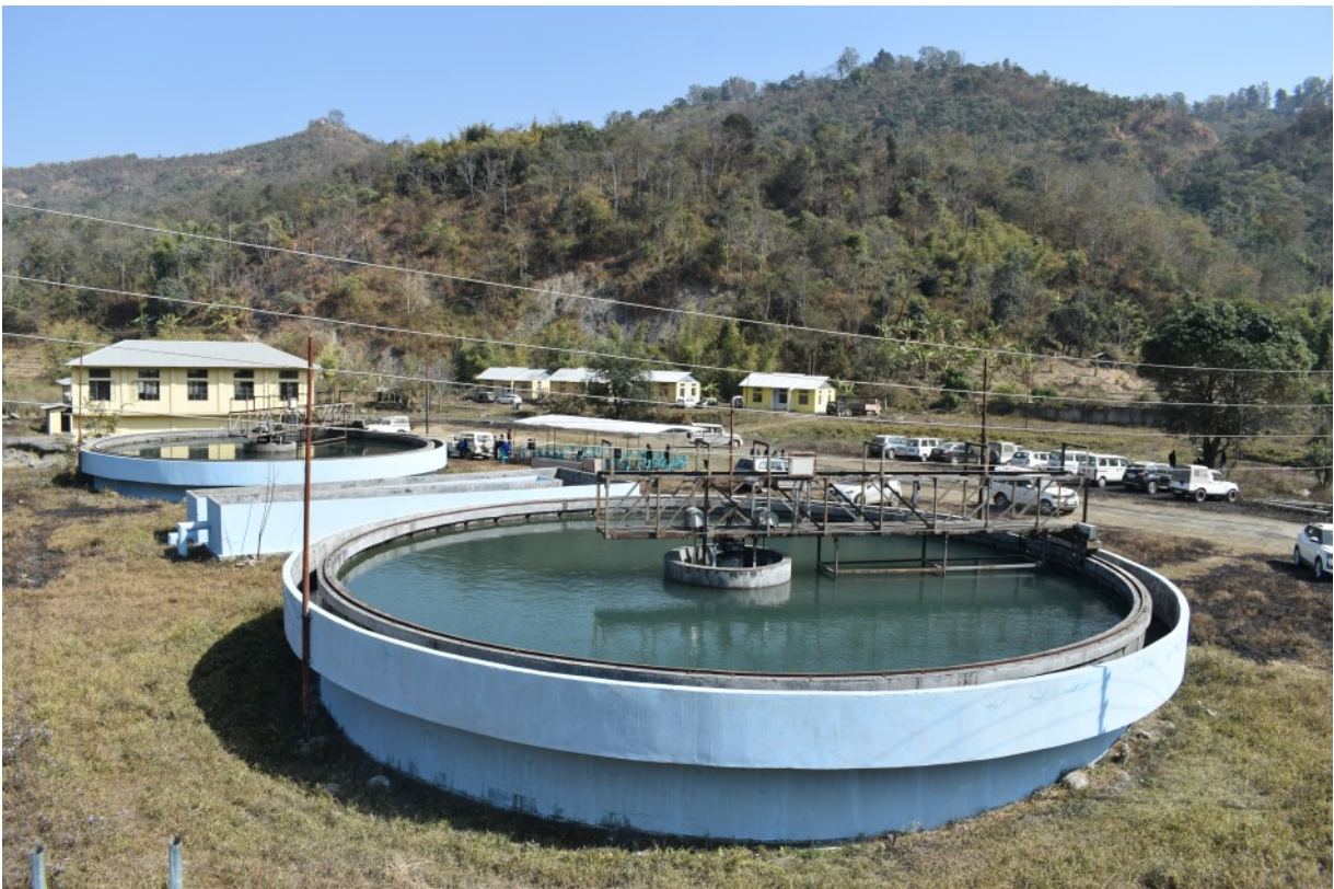
Sedimentation Tank at Water Treatment plant
