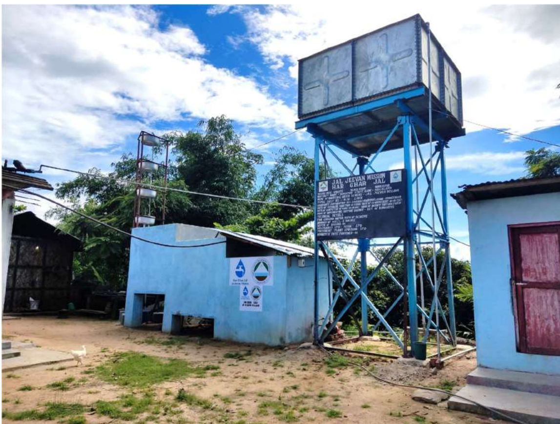
DEEP TUBE WELL WITH IRON REMOVAL PLANT WITH OVERHEAD GMS TANK AT VIHOTO VILLAGE, DIMAPUR
