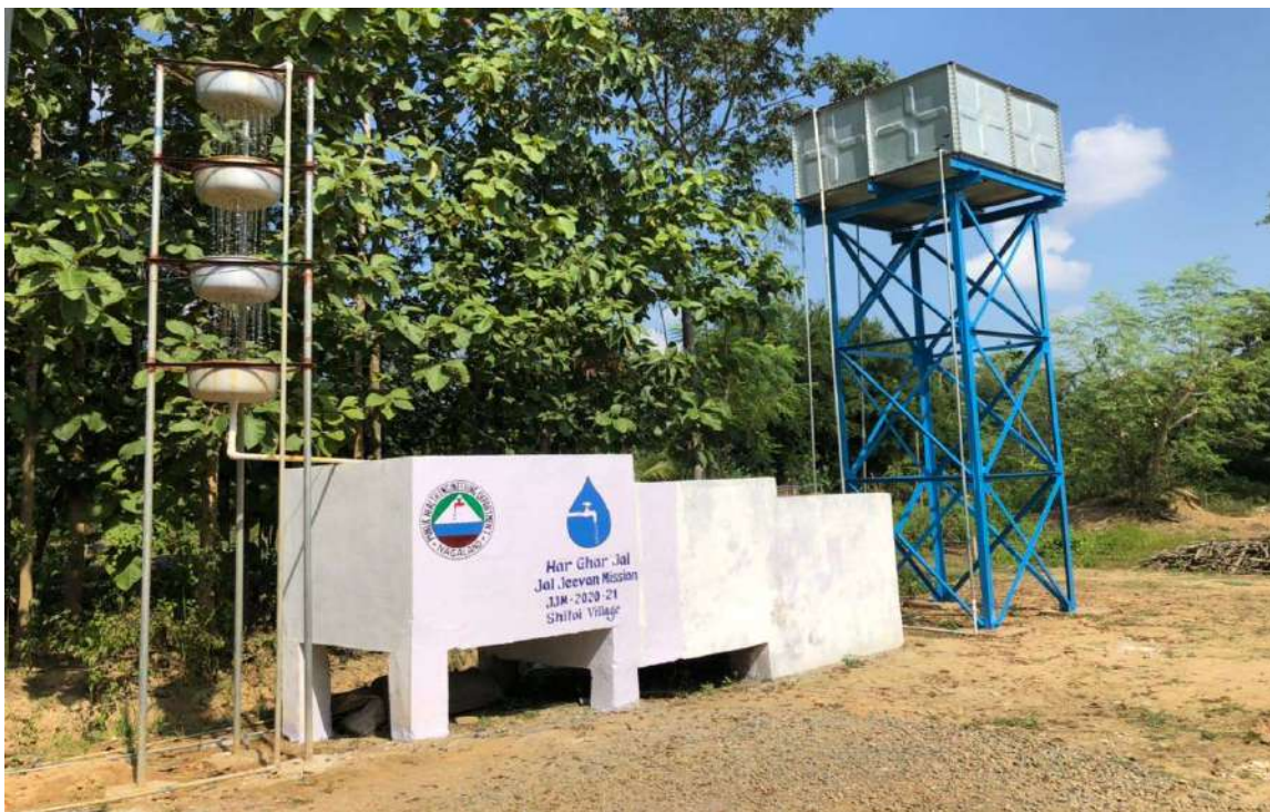
DEEP TUBE WELL WITH IRON REMOVAL PLANT WITH OVERHEAD GMS TANK AT SHITTOI VILLAGE, DIMAPUR
