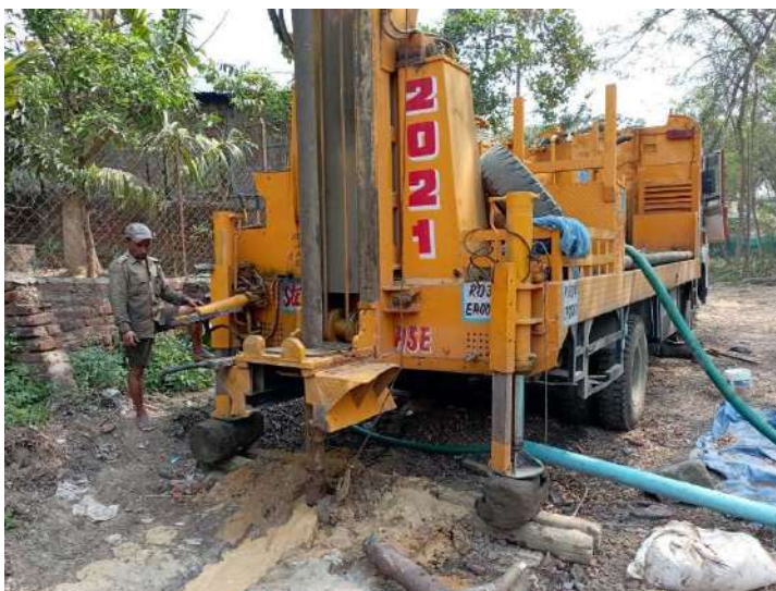
DRILLING WORKS FOR DEEP TUBE WELLS
