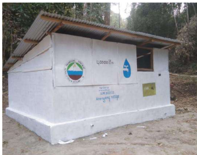
RCC MAIN RESERVOIR 40000 LITRES AT AMENYONG VILLAGE, MOKOKCHUNG
