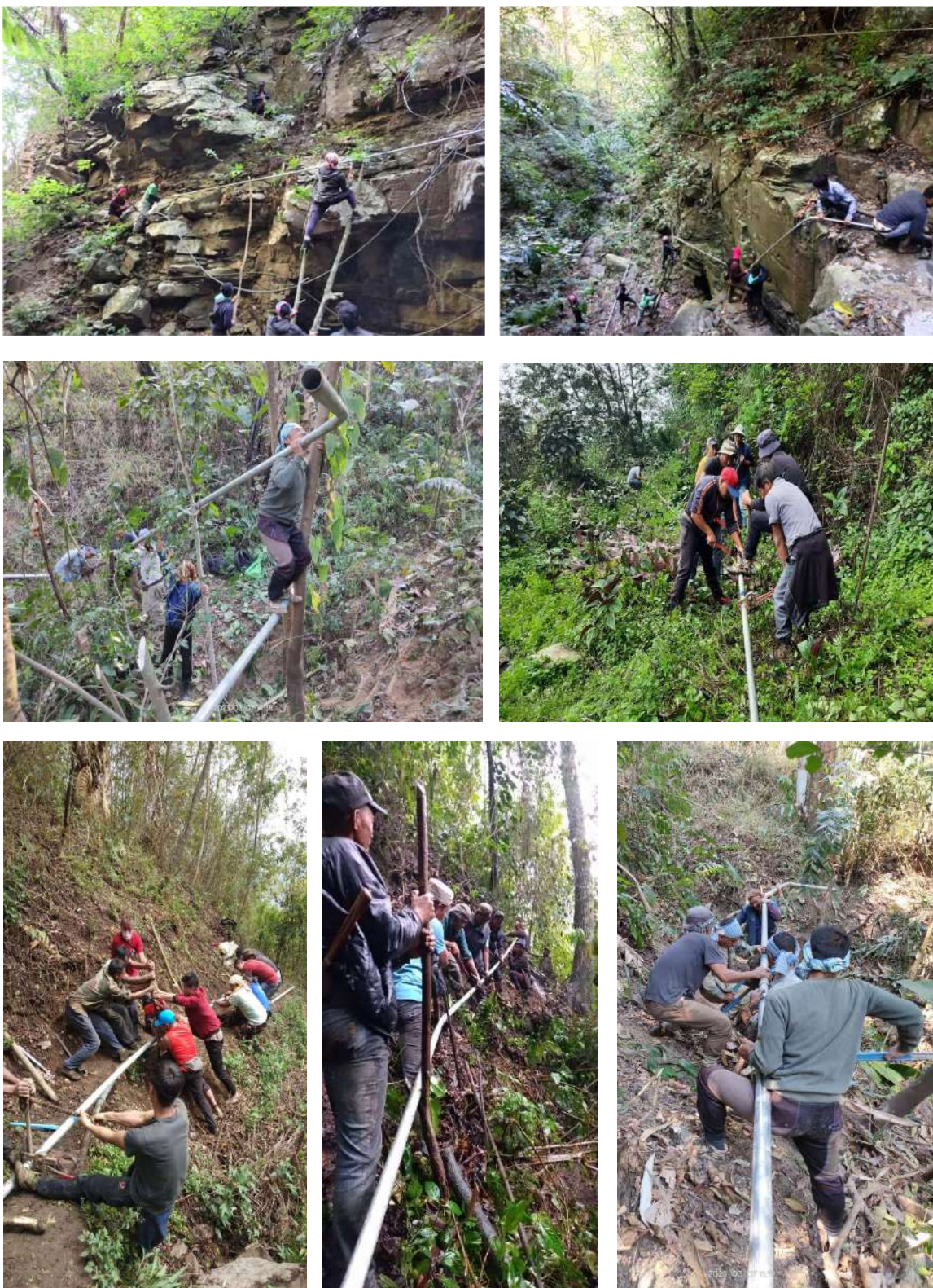
FITTING OF PIPES FOR JJM SCHEMES
