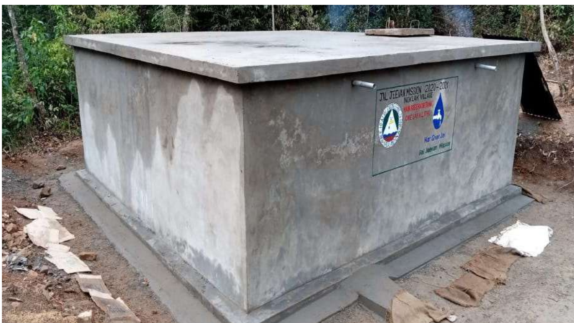
1 LAKH LITER RCC TANK AT NOKLAK VILLAGE, NOKLAK
