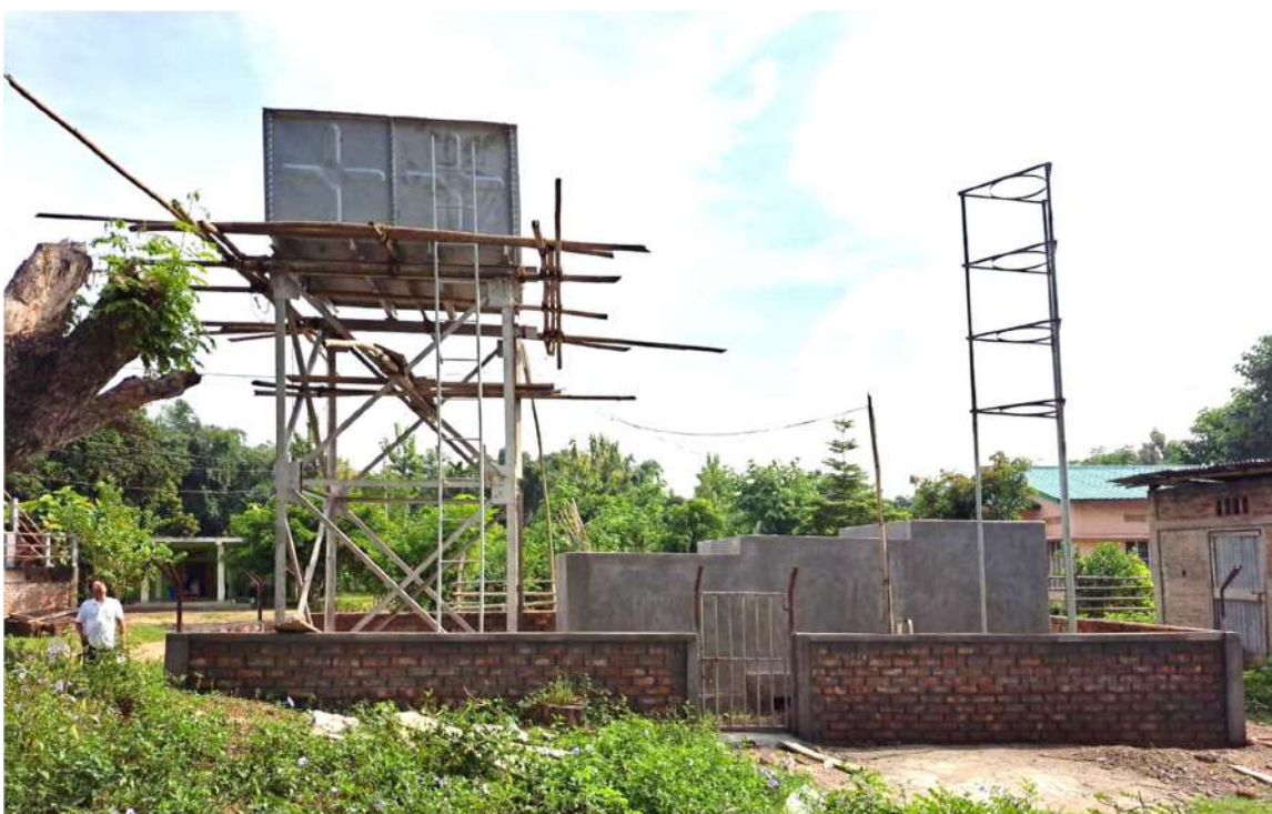
DEEP TUBE WELL WITH IRON REMOVAL PLANT AND OVERHEAD GMS TANK UNDER CONSTRUCTION AT NIHOTO VILLAGE, DIMAPUR
