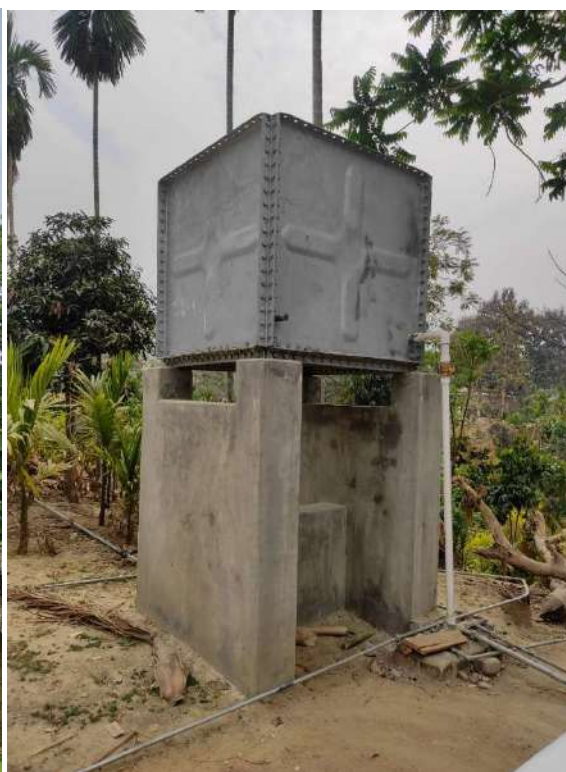
DISTRIBUTION TANK AT KHEHOI VILLAGE, DIMAPUR
