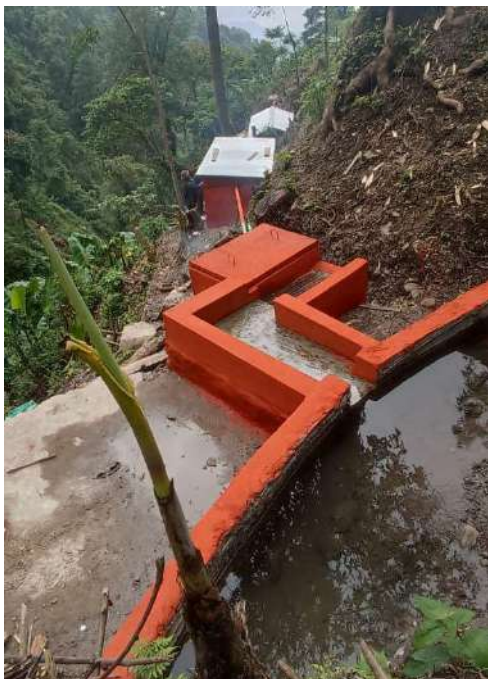
DIVERSION WEIR AND DESILTING TANK AT MONYAKSHU VILLAGE, MON
