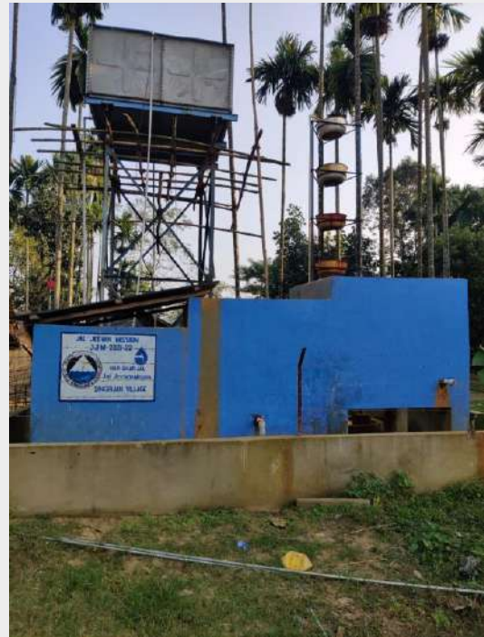
IRP WITH OVERHEAD TANK AT SINGRIJAN VILLAGE, DIMAPUR
