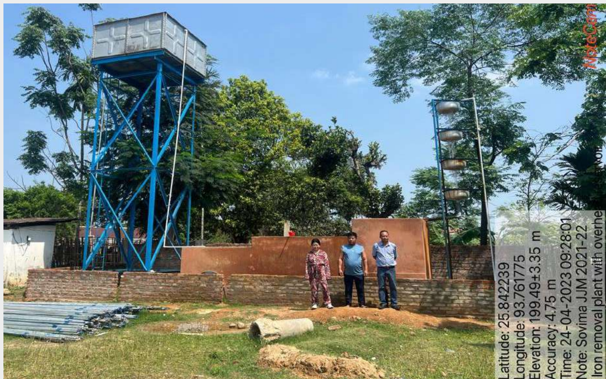
DEEP TUBE WELL WITH IRON REMOVAL PLANT AND OVERHEAD GMS TANK AT SOVIMA VILLAGE, DIMAPUR
