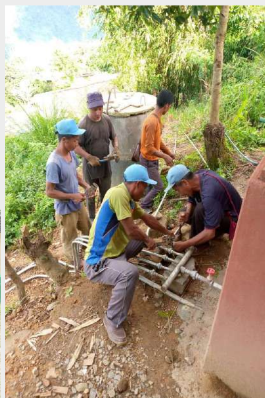
DISTRIBUTION MANIFOLD FOR FHTC CONNECTION
