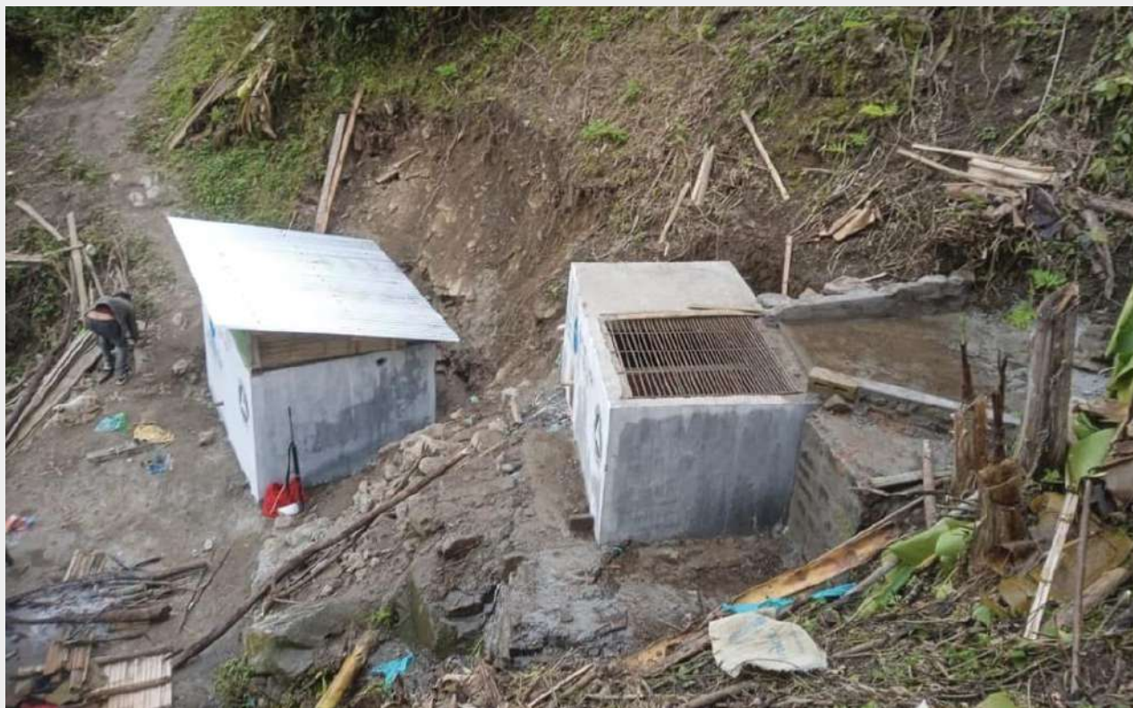
DIVERSION WEIR AND DESILTING TANK AT LUNTHUR VILLAGE, TUENSANG
