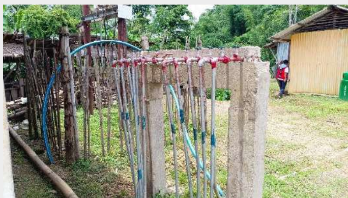
DISTRIBUTION MANIFOLD FOR FHTC CONNECTION
